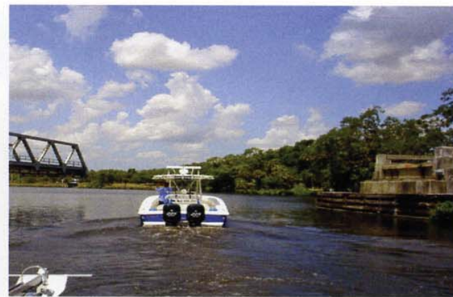
Approaching a rotating railroad bridge on the Okeechobee Waterway.
