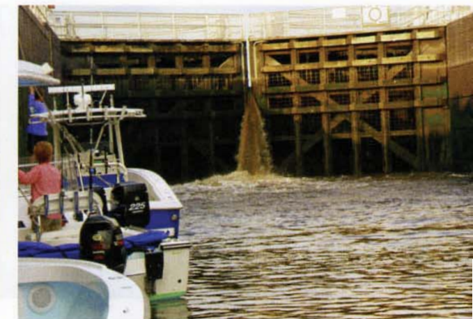
Inside the first lock of the trip, watching as the water level rises.
